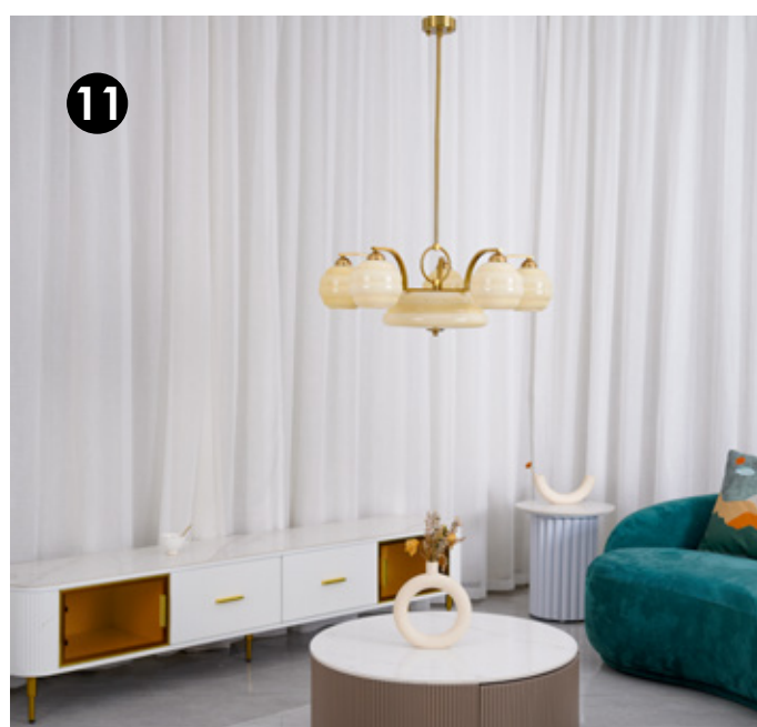
Installed and fixed to the ceiling
